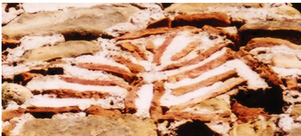
Fig. 61. Angelokastro, SW building, W façade, tree of life in the masonry.
